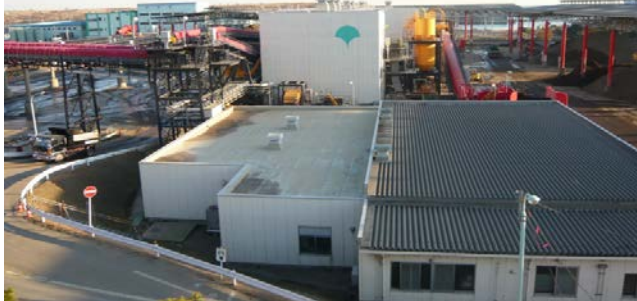
Main Building of Tokyo Metropolitan Construction Waste Soil Recycling Center (Source: Center's Brochure)
