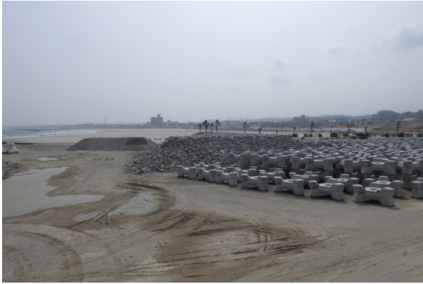
Sea Dike Reconstruction Project in Iwaki city
