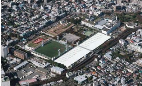
Ochiai Water Reclamation Center
